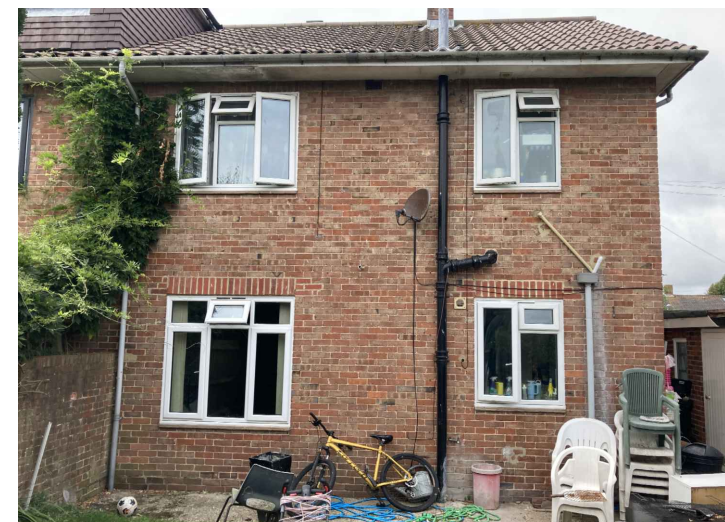
Photo 2: Existing rear elevation
