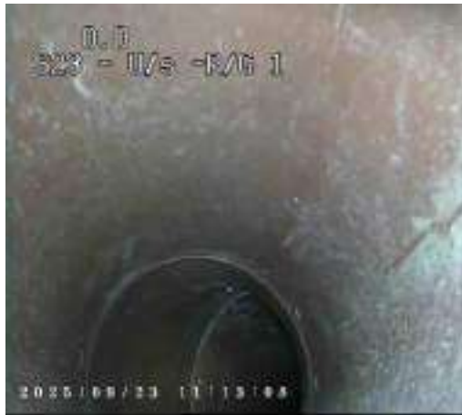
874238e3-5c8d-4e62-b337-53ff713bc800.png, 00:00:01, 0.00 m Start node, manhole, reference: S23
