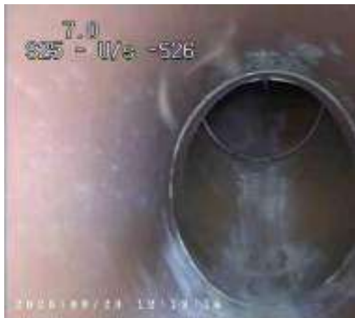
5ab9e6b5-f018-4830-aeaf-59413b88e469.png, 00:00:55, 7.00 m Line deviates up
