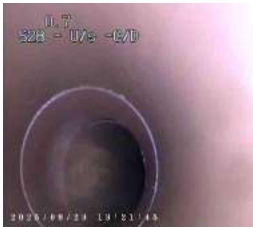
a825371b-8433-4ff9-8a59-269a2f0f1fb1.png, 00:00:04, 0.70 m Line deviates right
