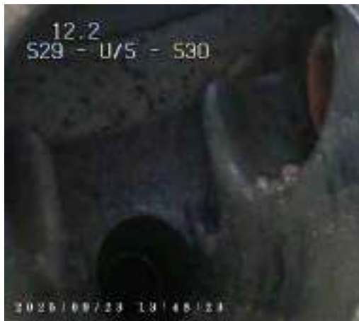
f6364dc1-c979-467a-b580-27cc55d3978c.png, 00:00:48, 12.20 m Finish node, manhole, reference: S30
