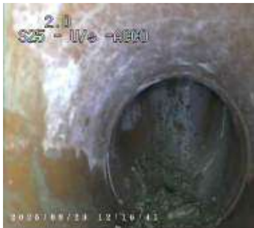
04b3d232-ea49-45fd-9245-83eb565c9aeb.jpg, 00:00:13, 2.00 m Line deviates up
