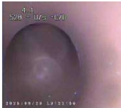
ed2bbe49-3a52-4504-ada8-2e9e5e607fa5.png, 00:00:16, 4.10 m Line deviates up
