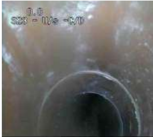
9f1f96d6-ed85-486c-a8cb-51220865b82c.png, 00:00:00, 0.00 m Start node, manhole, reference: S23
