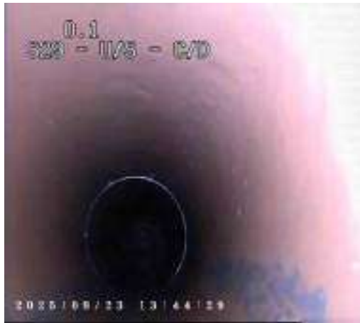
5519ed24-8b40-4765-8877-b93eeaf4e504.png, 00:00:00, 0.00 m Start node, manhole, reference: S29
