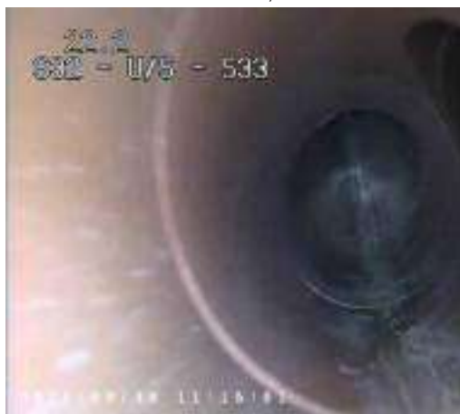
98dac559-fbb3-446c-908e-08fb8c5f31e0.png, 00:02:13, 22.20 m Junction at 2 o'clock, 100mm dia
