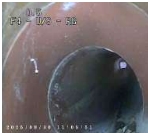
2e142608-22fa-4c6f-8e6b-37d59d3e7981.png, 00:00:03, 0.50 m Line deviates right
