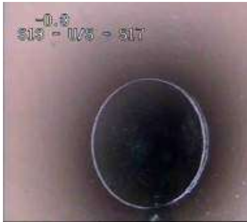
90942ca6-c72b-43cb-b74f-7ce43157ffce.png, 00:01:10, 0.00 m Start node, manhole, reference: s13
