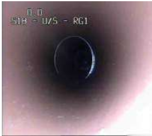
7bff1beb-0aba-4fca-8118-210864cef42e.png, 00:00:00, 0.00 m Start node, inspection chamber, reference: S18
