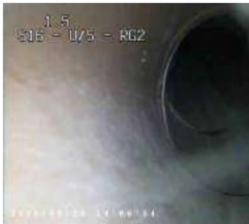
90d6bf2f-bee8-49c9-8be4-2fe3fc35f5ca.png, 00:00:09, 1.50 m Line deviates up
