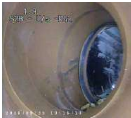
570285eb-0149-4694-9a15-2caf9bfe6580.png, 00:00:07, 1.90 m Line deviates right
