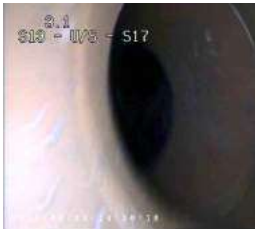
c7373a10-6427-4a1d-b77a-5ff050277d97.png, 00:00:12, 3.10 m Line deviates left
