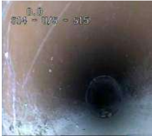
d547f25a-5a35-4550-abcb-101c80ee385a.png, 00:00:00, 0.00 m Start node, manhole, reference: s14
