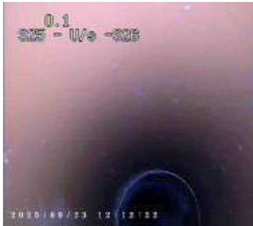
448cd648-26ed-4884-9719-0c7437a317c6.png, 00:00:00, 0.00 m Start node, manhole, reference: S25
