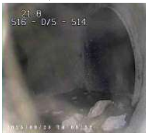
4235ffb7-4764-42d1-8123-ed97d289eccc.png, 00:00:52, 21.80 m Finish node, manhole, reference: s14
