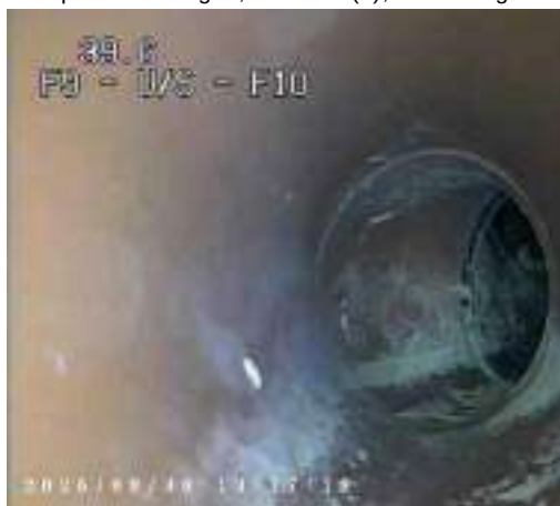
688b7e48-5183-4e84-b0e0-9d8210ba43bb.png, 00:03:31, 39.60 m Line deviates right
