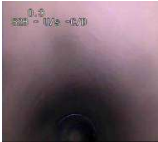
4a9f9f6a-40dc-474e-9dba-249349e5ecb3.png, 00:00:01, 0.00 m Start node, manhole, reference: S28
