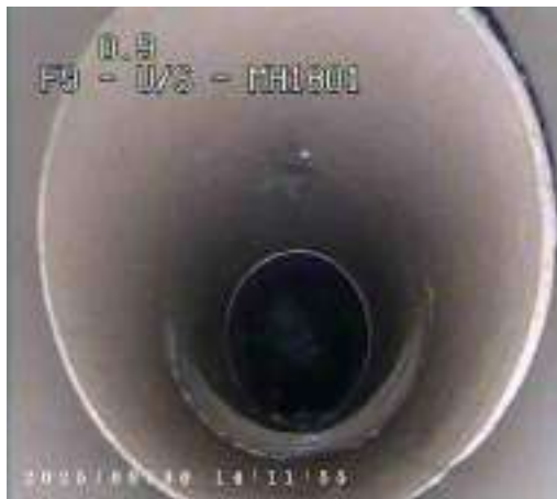
e0b41bd5-bc86-4dce-9882-5db932d9bc49.png, 00:00:07, 0.90 m Junction at 6 o'clock, 150mm dia, from back drop
