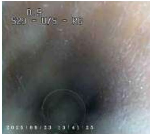
86bb7a12-c139-46a8-b735-9561efe057c5.png, 00:00:01, 0.00 m Start node, manhole, reference: S29
