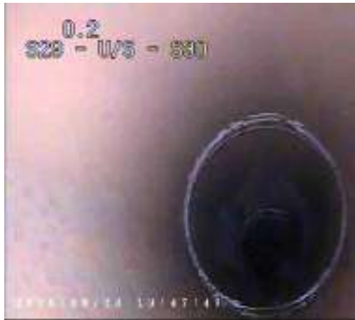
552225ef-6894-4408-91b7-d4918a7fce2d.png, 00:00:13, 0.00 m Start node, manhole, reference: S29
