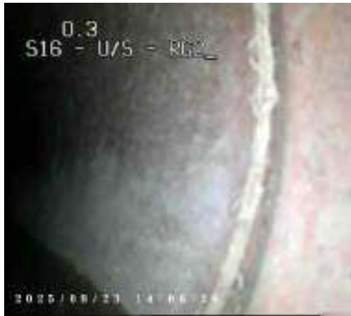
0d5195b4-c784-4ab6-849a-35595ee2415c.png, 00:00:00, 0.00 m Start node, manhole, reference: S16
