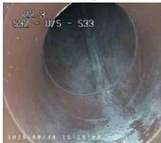
bdb046af-d0c2-4190-9d11-a8424960e074.png, 00:02:14, 22.30 m Line deviates up
