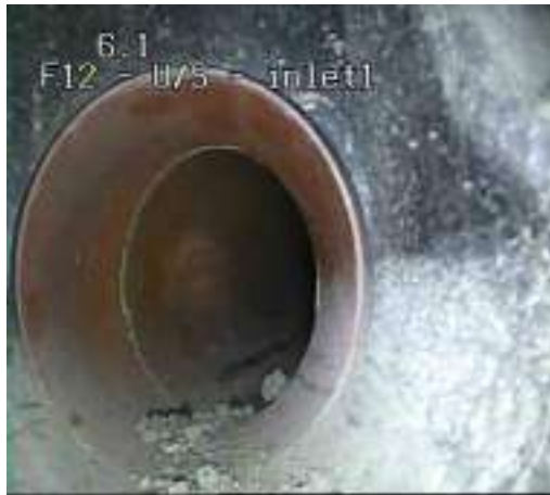
5d2f881f-b17b-4b4f-a1bf-4f925f39d540_1.png, 00:00:01, 0.00 m Start node, inspection chamber, reference: F12
