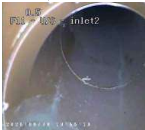
b1e89e72-83e0-43ff-b684-b396c60adff3.png, 00:00:04, 0.50 m Line deviates up
