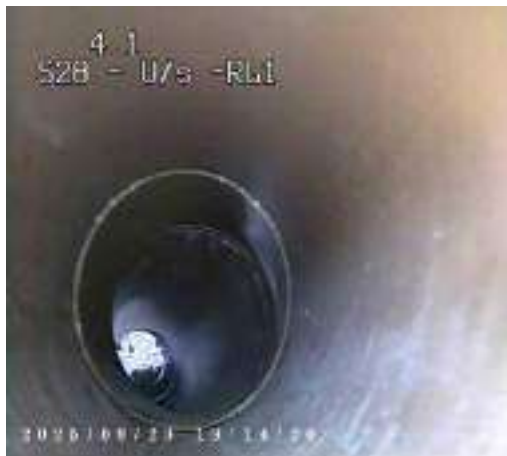
db528742-4aa7-45b8-9fc9-7131d8da503e.png, 00:00:15, 4.10 m Line deviates left
