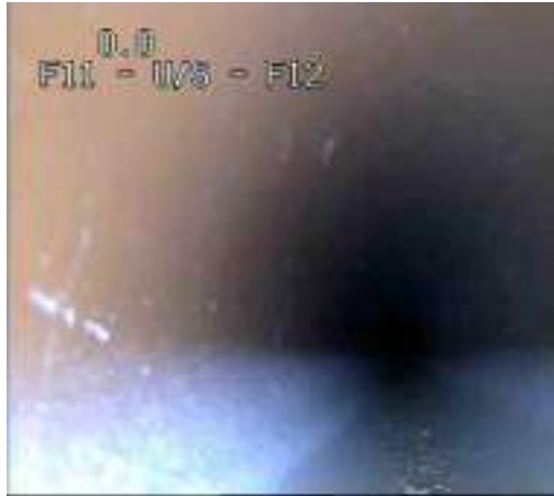
f2b8818c-1d2a-4039-91dc-20dc7210c3b9.png, 00:00:00, 0.00 m Start node, inspection chamber, reference: F11
