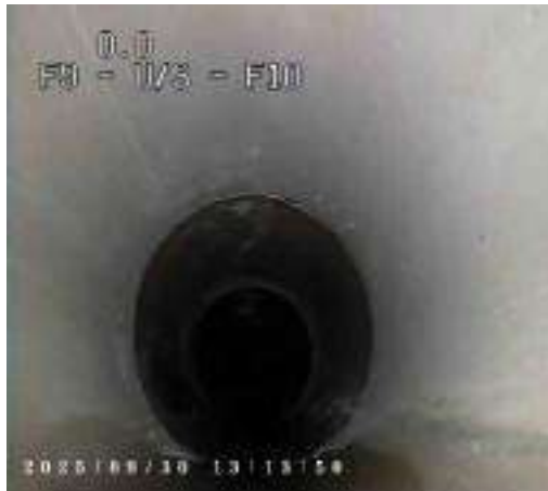
f7eba1e0-3961-44d8-bae5-55cd0b907470.png, 00:00:03, 0.00 m Start node, manhole, reference: F9
