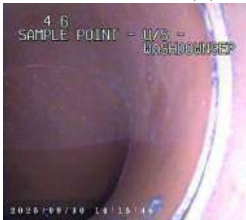
74be748c-f2ad-4be4-8b77-743ea1818809.png, 00:00:14, 4.60 m Line deviates down n
