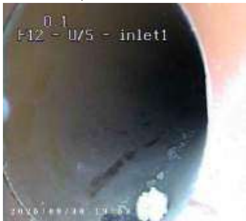
5fb6379b-8aed-4e8a-9108-1637e9d32eb4.png, 00:00:05, 0.10 m Line deviates right
