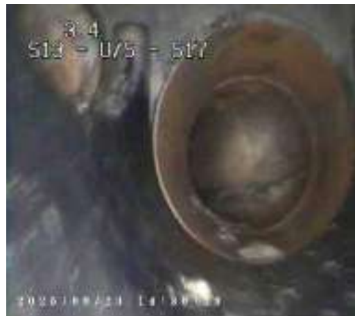
84b899c3-899e-4676-9b82-a2a593a5b3e0.png, 00:00:13, 3.40 m Finish node, manhole, reference: S17
