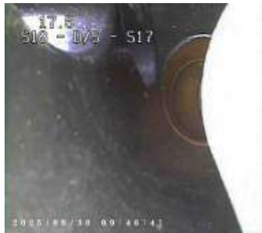
dc8405d8-ca1a-459c-a41d-3600236bc006.png, 00:02:05, 17.50 m Finish node, manhole, reference: S17
