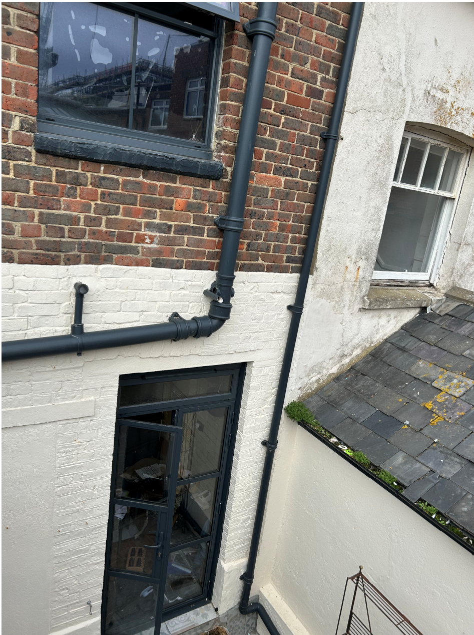
Existing rear elevation viewed from second floor terrace
