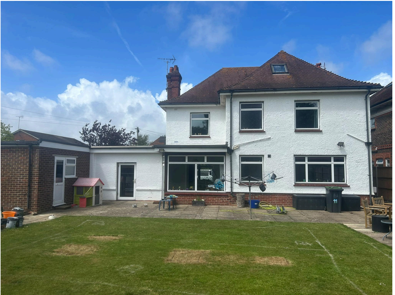
Image 2: view from rear garden towards house
