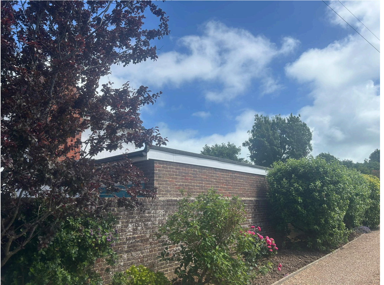
Image 10: view of existing garage
