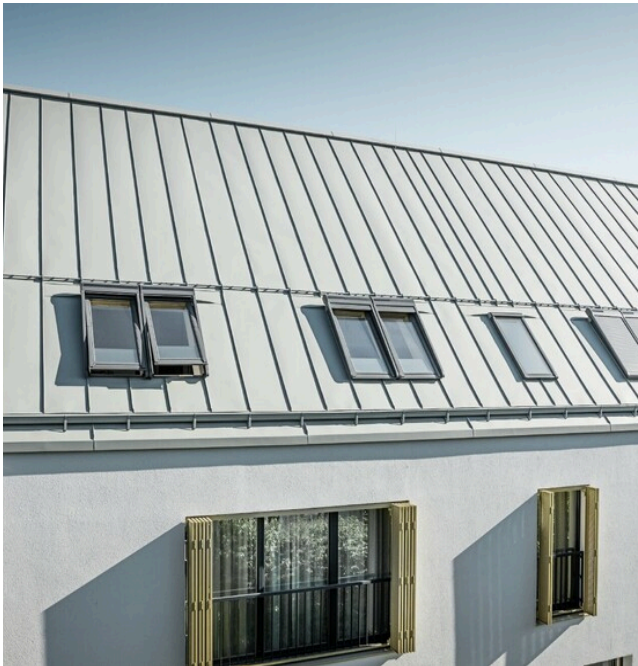
Rear Extension, Garden Room and Dormer Roof: Metal standing seam in light grey
