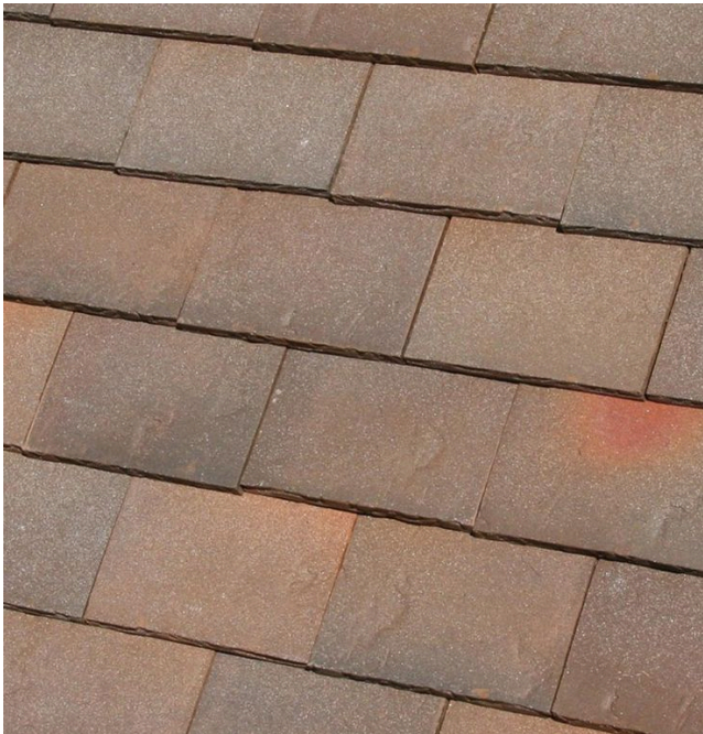
Side Extension and Replacement Roof Finish: Plain tile roof
