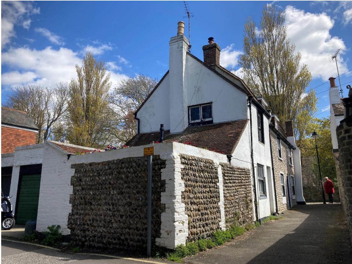
Image 04 – No. 2 & No. 1 Old Swan Cottages viewed from Middle Street looking North-East
