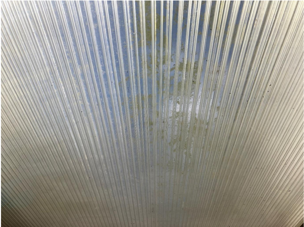
Image 08 – Polycarbonate roof viewed from inside
