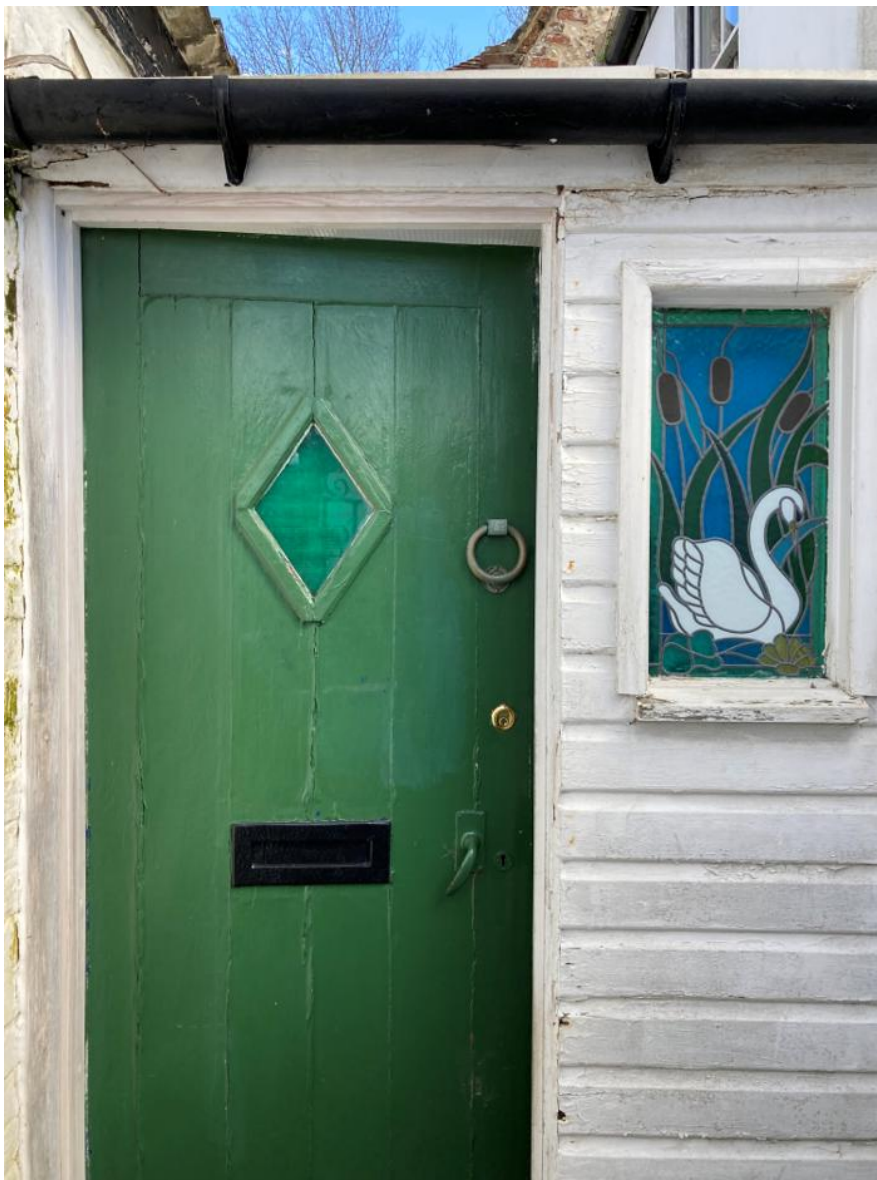
Image 06 – Existing front door, stained glass window and timber cladding.
