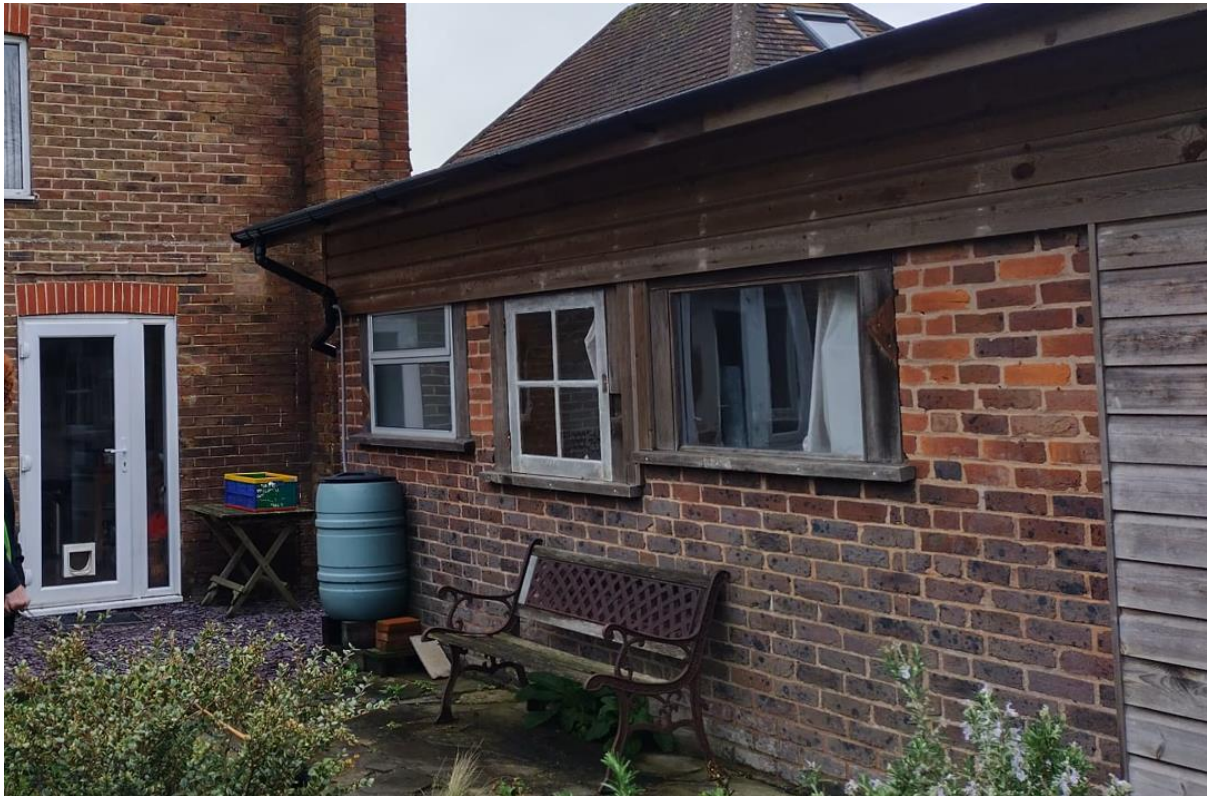
Figure 1: The outbuilding, showing the close relationship with the main house on the left
