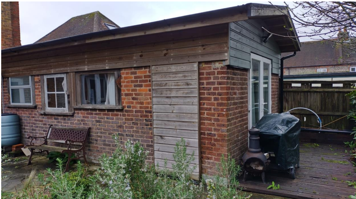
Figure 2: Rear elevation, leading to small timber deck for sitting out
