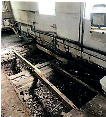
Rotten floor Joists and infested with dead and live Rats. Drain outside the kitchen, again many years of neglect and lack of maintenance. Environmental health nightmare.
