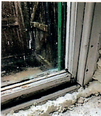
kitchen window which is completely rotten and loose, commercial extractor vent in very poor state and broken.
