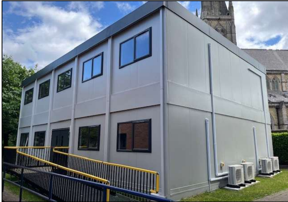
Figure 6 Example of a single two-storey Modular unit
