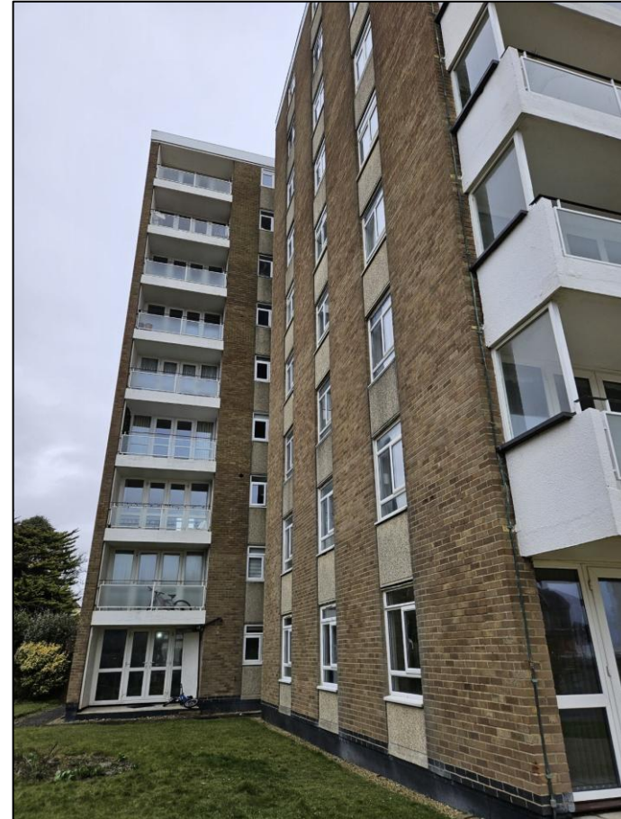
Figure 9 Existing External Wall
