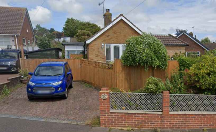
③ Boundary fence corner plot - 49 Cleveland Road
