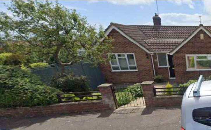
① Boundary fence corner plot - 64 Cleveland Road
