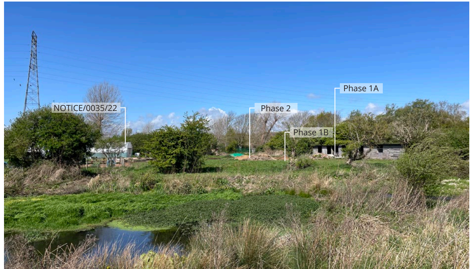
21 View from the east boundary of the site looking west.
