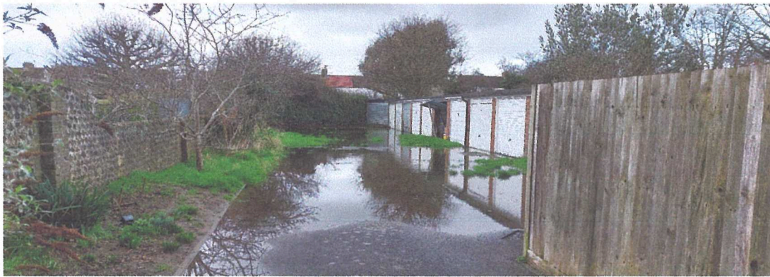
Garages between Southview Road and Underdown Road, adjacent to the site of the proposed development, and built on the water course of the old brook. Photographed week commencing 23 rd February, 2026
