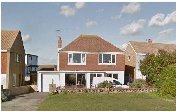
Front and west facing side of House
