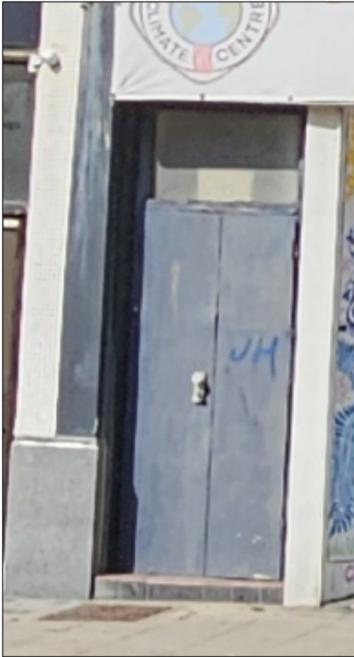
Door ED02 as Existing Photograph
