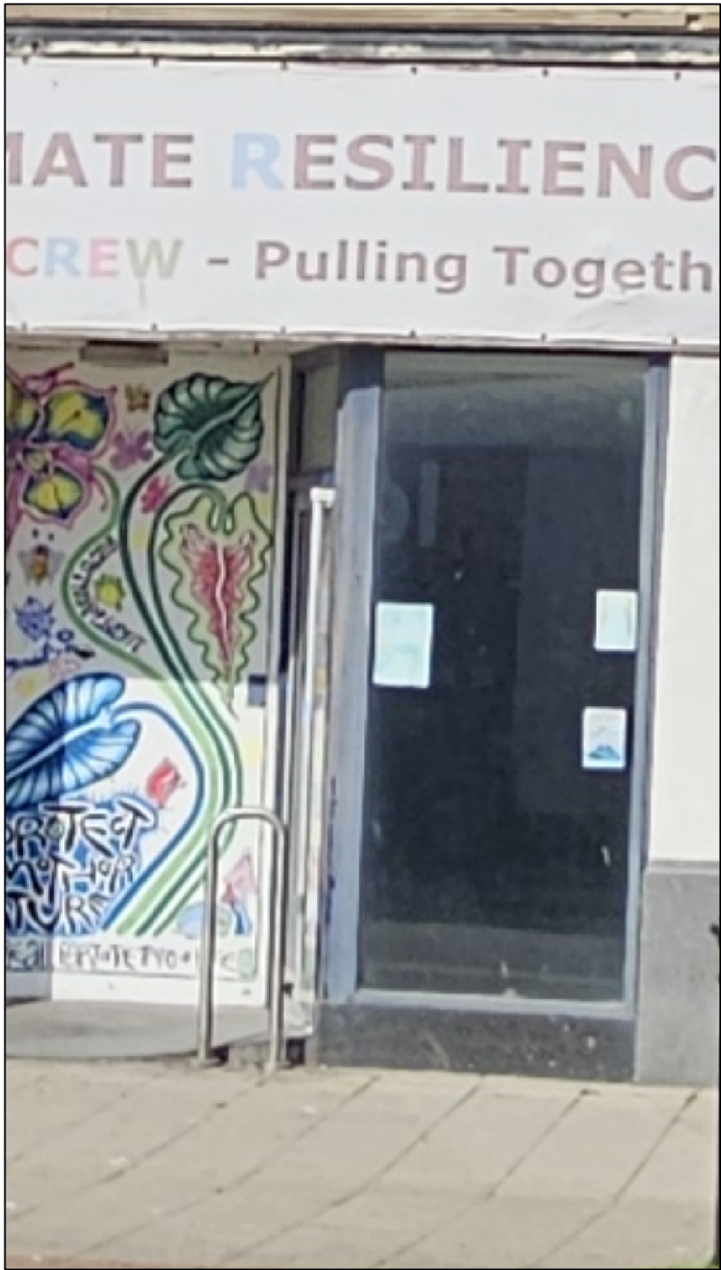
Shop window GW02 & door ED01 as Existing Photograph
