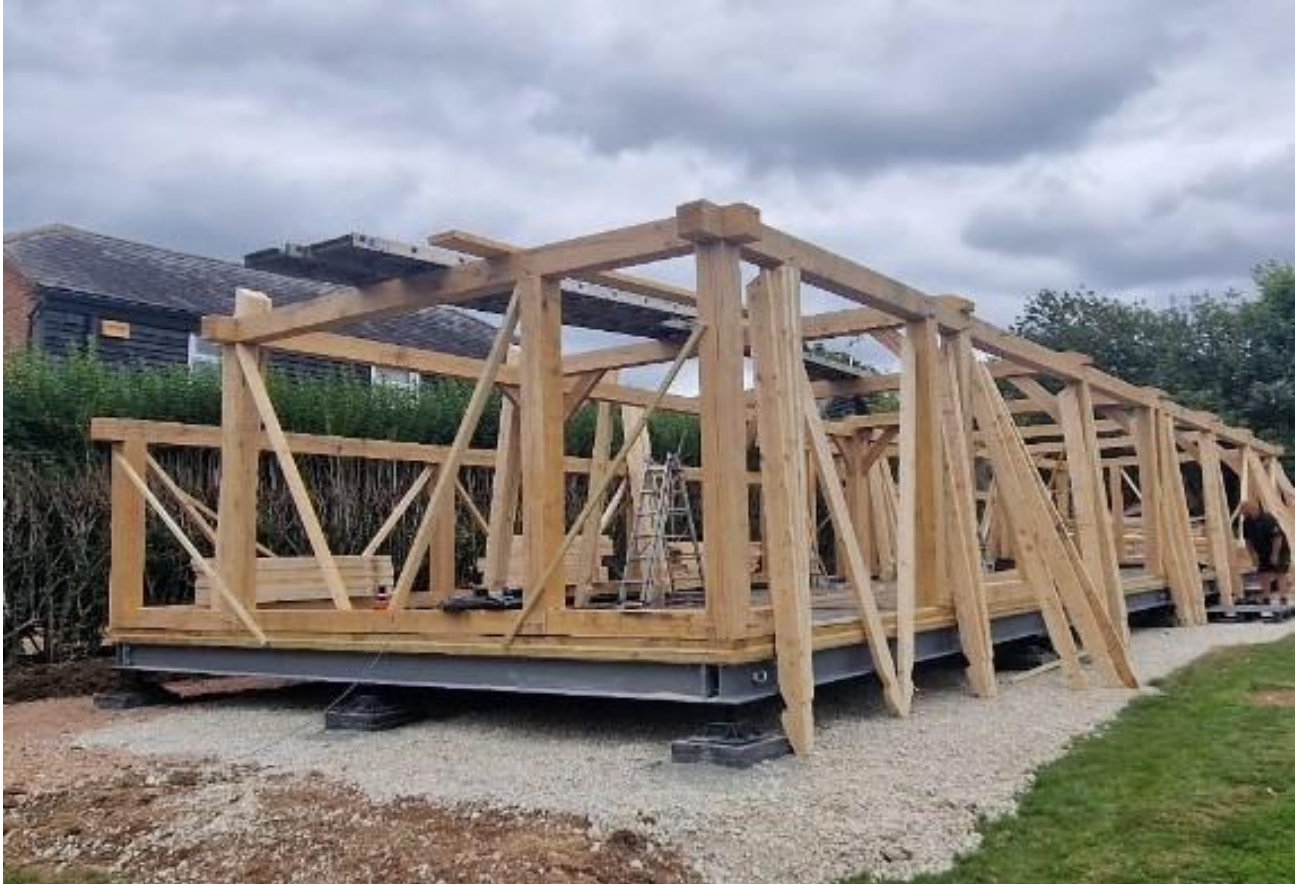
Examples of steel chassis upon which the caravan will be sited:
