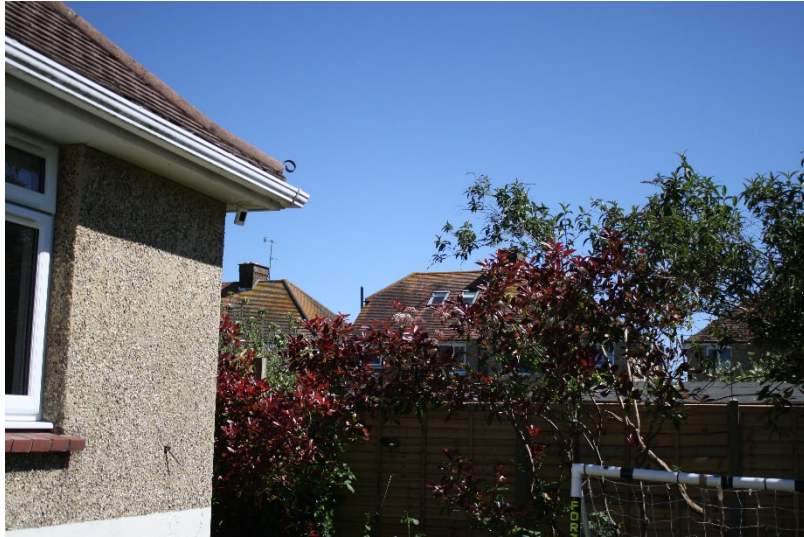
Rooflights to rear of 37 Haynes Road, facing rear of house
