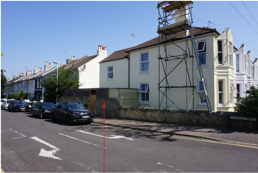
Existing side extension to be replaced.
