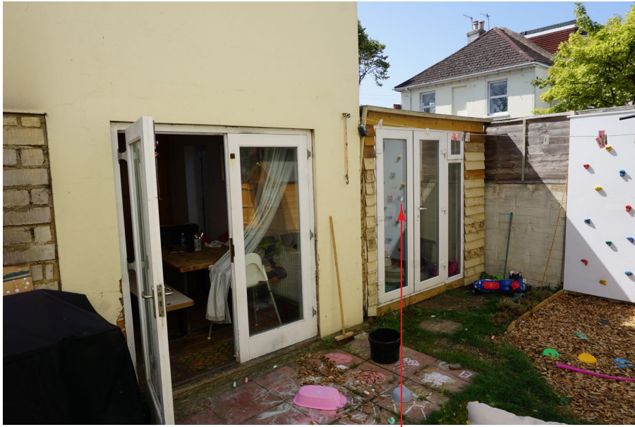
Existing side extension to be replaced.
