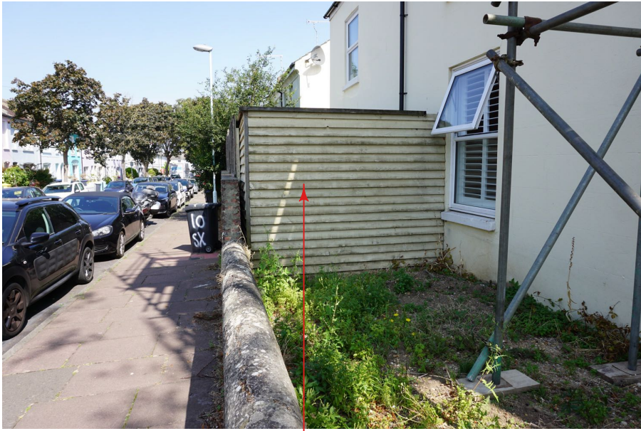
Existing side extension to be replaced.
