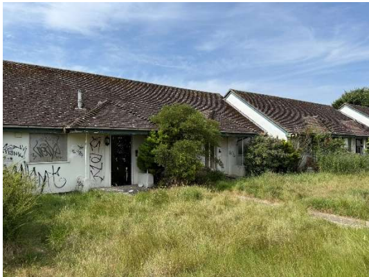
Photo 7: General View of Building 2.
