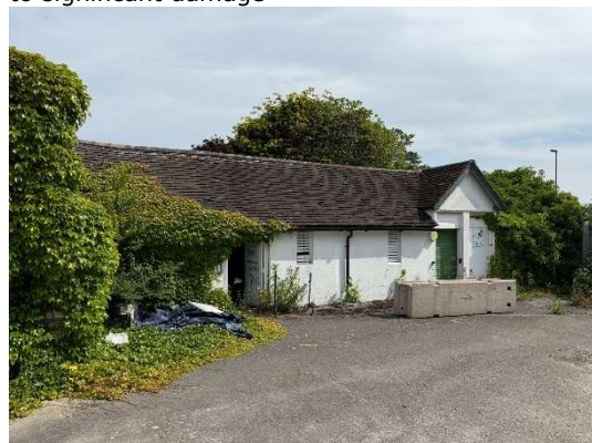
Photo 6: General View of Building 1
