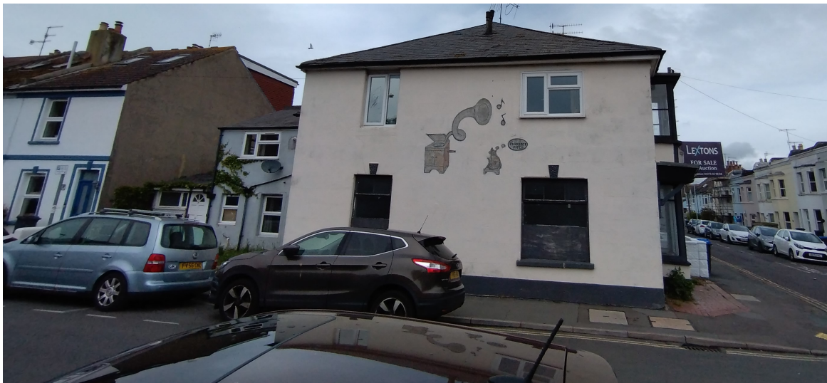
View from Anglesea Street
