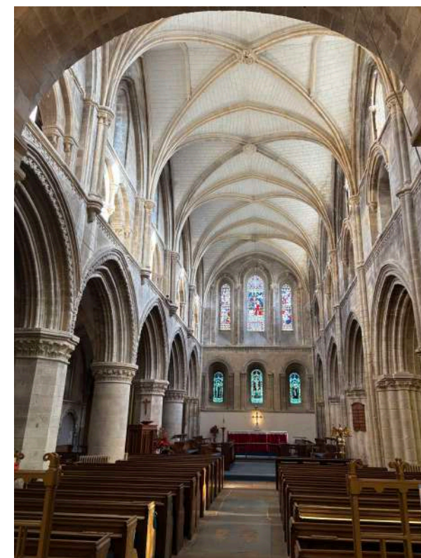
Nave of the Church illustrating the differences in architectural style and detailing
