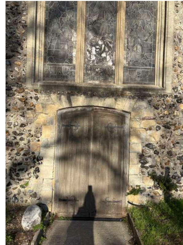
Existing timber door and access to south transept
