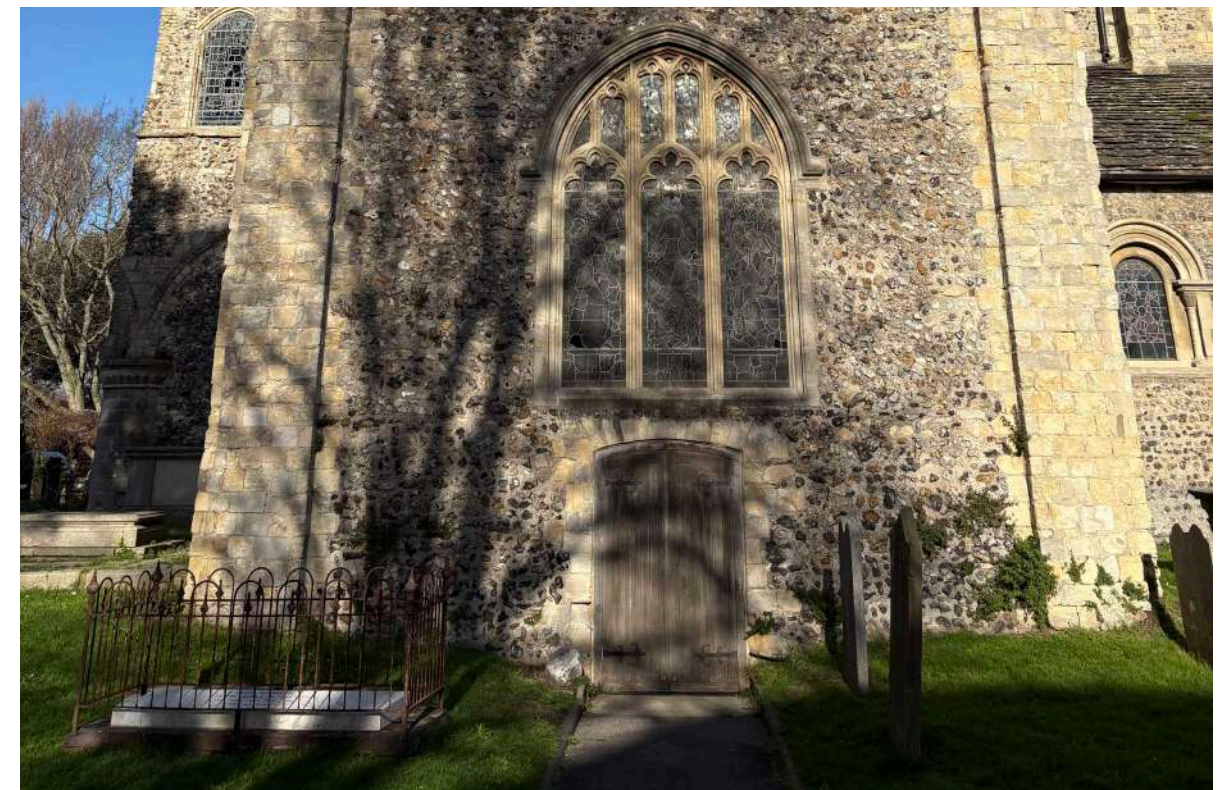
South elevation of south transept and existing gravestones and railings in churchyard
