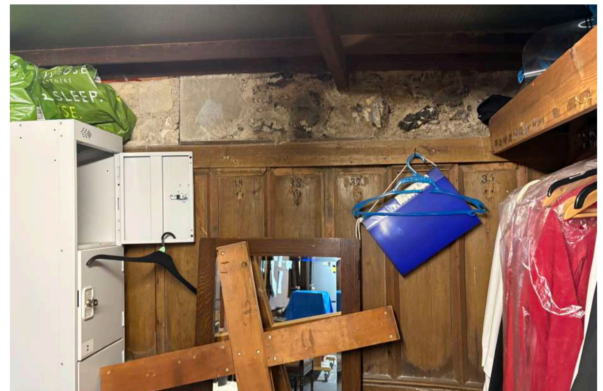
Earlier timberwork within the vestry, adjacent to stonework
