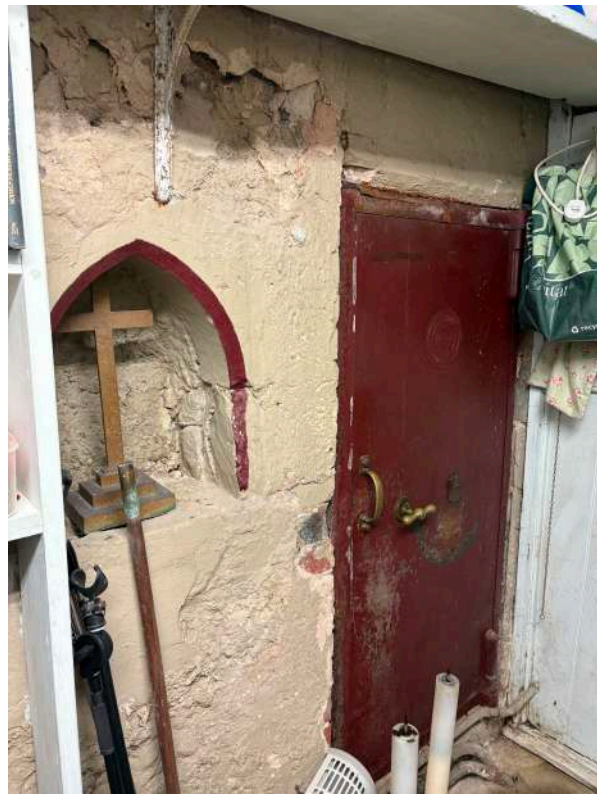
Medieval piscina set in the stonework of the south elevation of the south transept (vestry office), with a safe to the west
