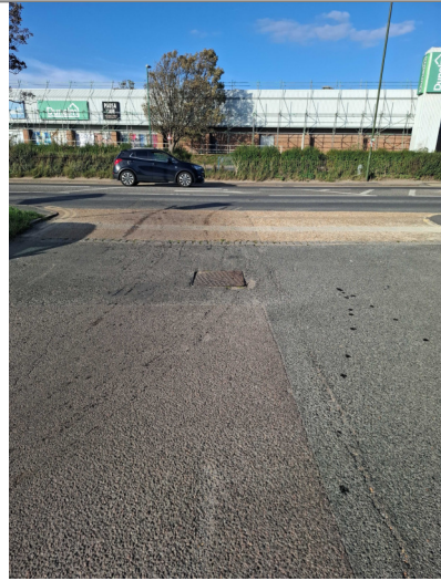
Other Site Photos: SWMH-1
