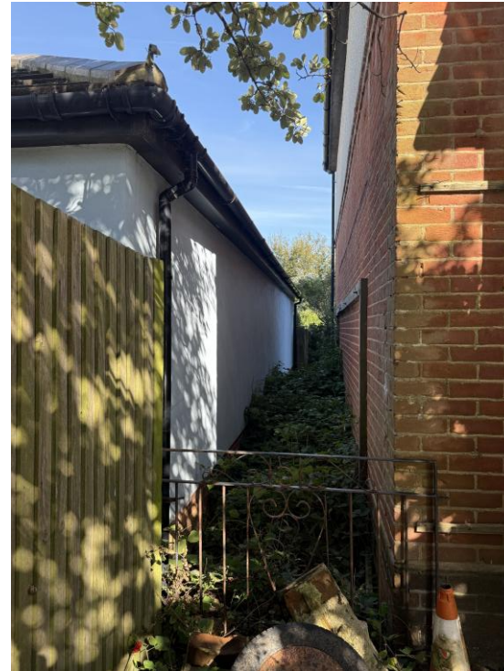
Figure 3 View of Side elevation to No.30
