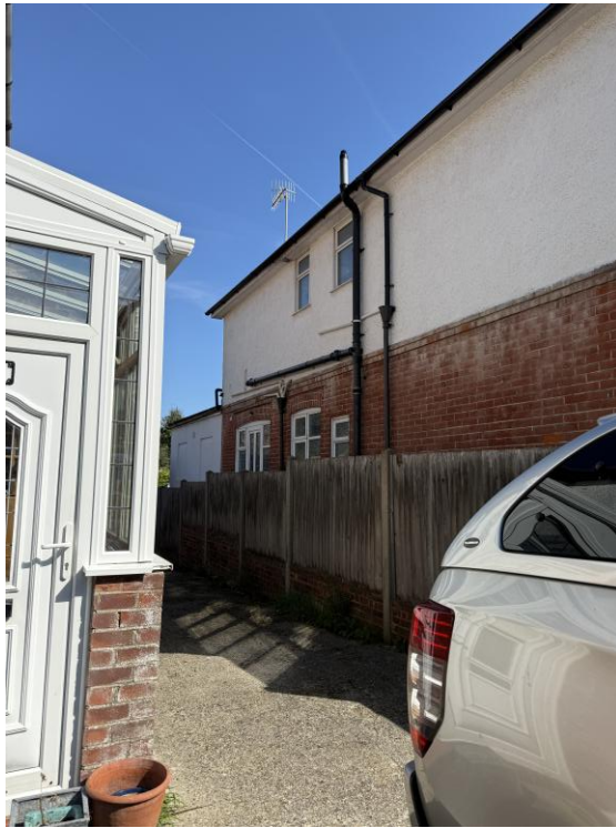
Figure 2 View of No.26. side windows. All obscured glazing and utility spaces
