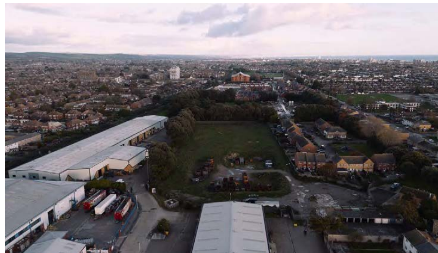
2. VIEW FROM THE WEST
