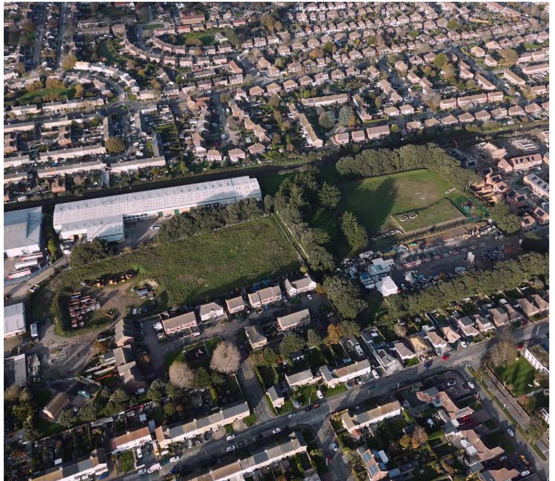
DRONE SHOT OF SITE
