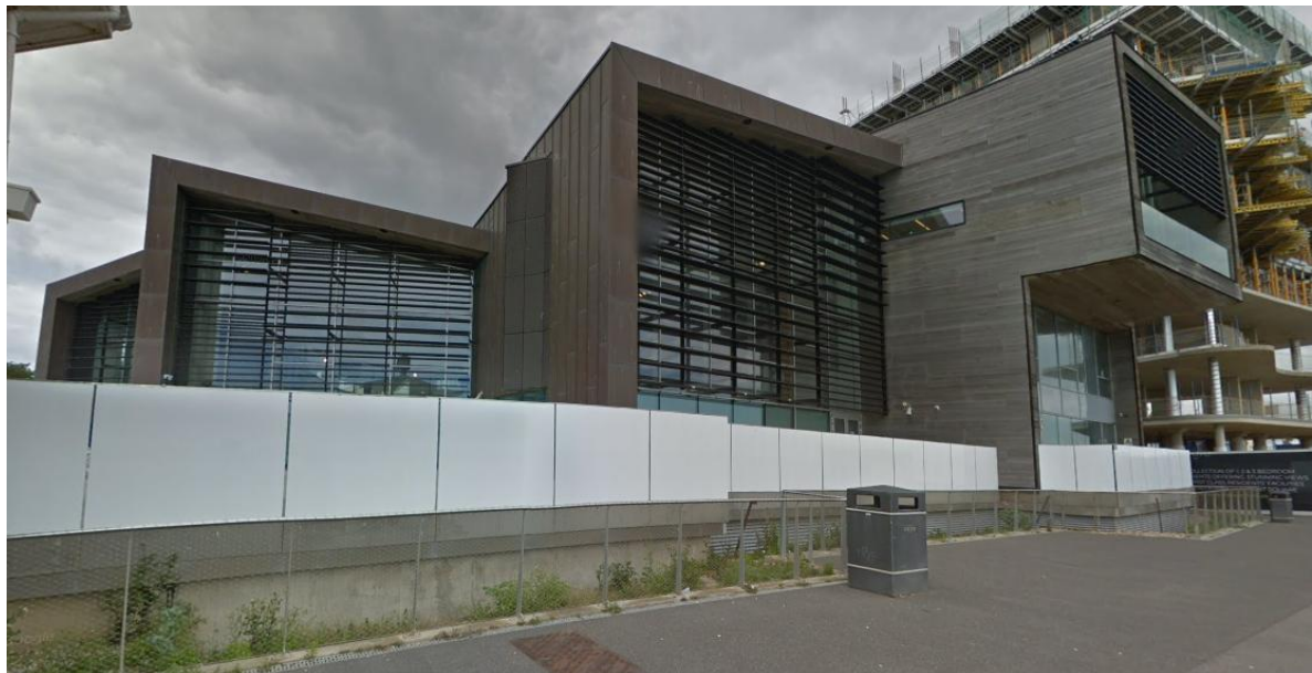
Figure 2: Obscured Balustrading to Splashpoint
