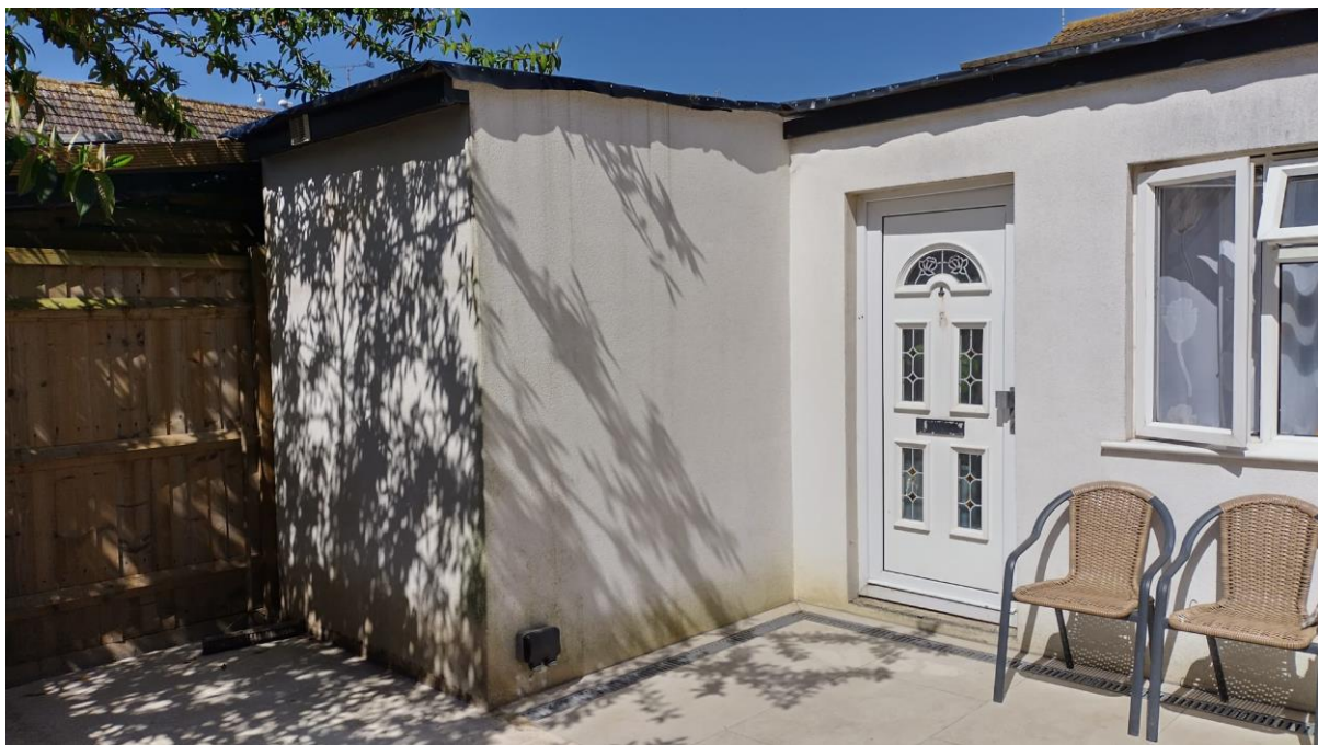
Figure 2: The small extension forming the shower room
