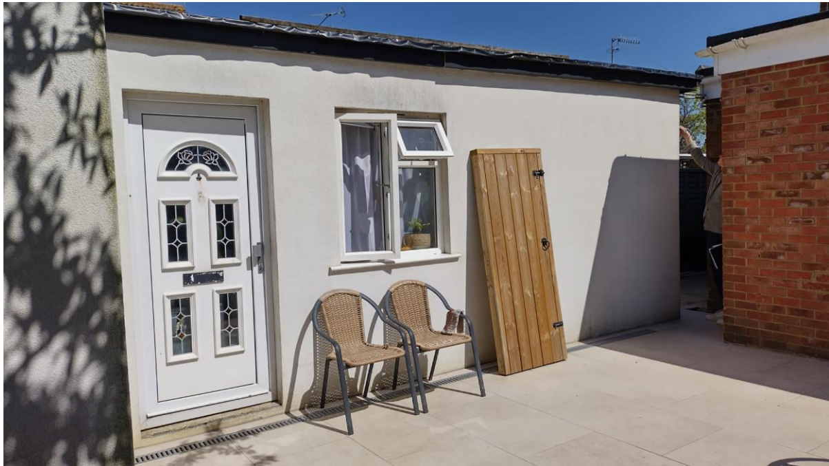
Figure 1: The annex. The house extension is the brick structure on the right hand side
