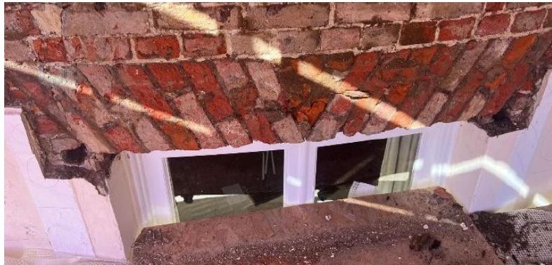
Figure 5: Soldier course lintel above window
