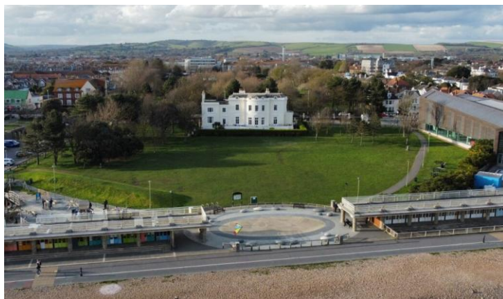
Figure 2: Overview of Beach House relative to its surroundings
