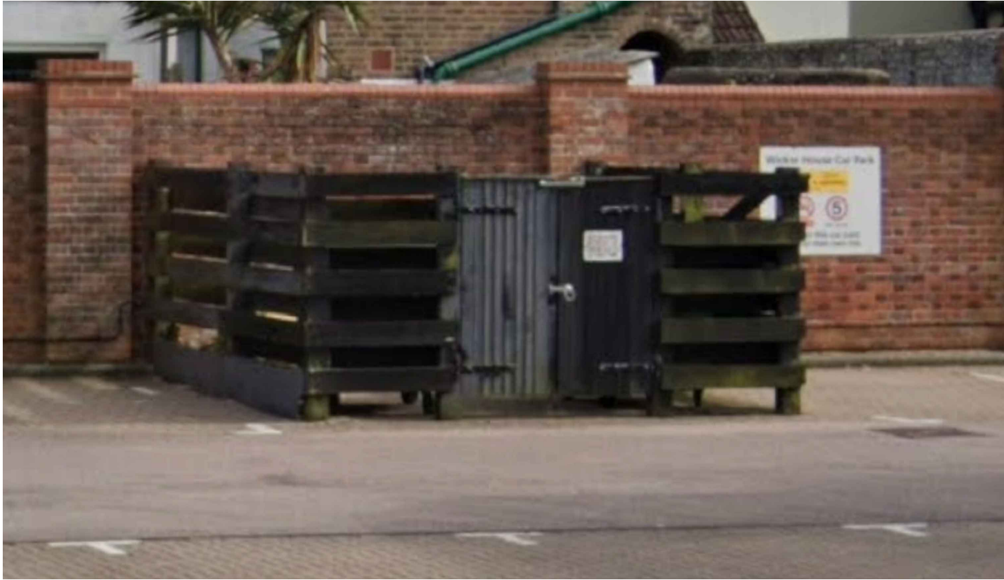
New bin store to match existing bin store on-site
