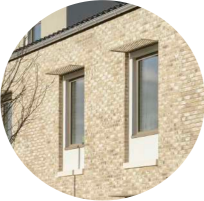
D: Glazing ratios balance daylight and overheating. Solar shading and openable windows help regulate temperature.
