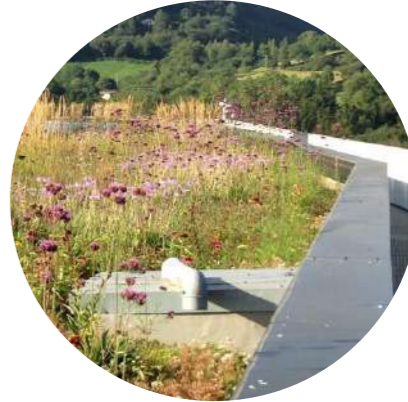
F: Green Infrastructure. Provision of green roofs and retention of existing planting assist with biodiversity net gain and ecological benefits.
