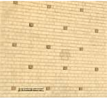
Materiality of existing presbytery - light buff brick
