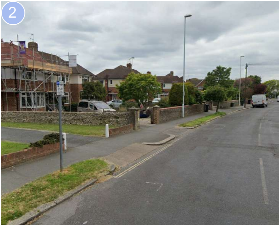
Looking west along the south side of Chesswood Road
