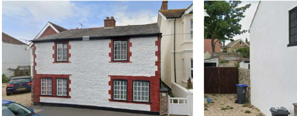
Old Mill Cottage and side walls to rear garden - Grade II
