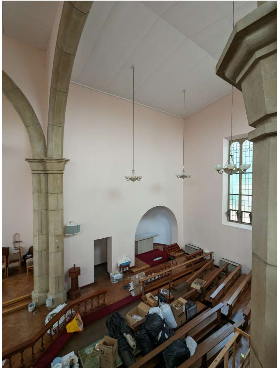
view from the mezzanine looking towards the east transept
