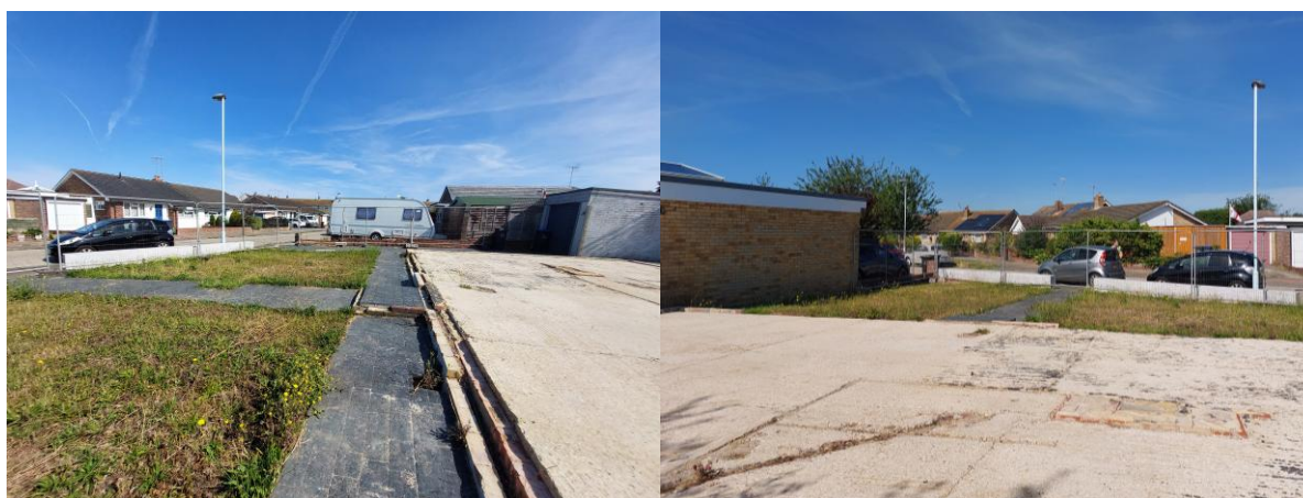
Image No. 02 & 03 – Hardstanding pavement leading to prior property (left) and hardstanding foundation of prior property (right).
