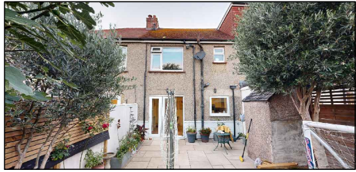
REAR ELEVATION PHOTOGRAPH
