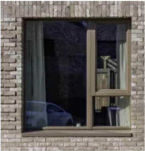
4 High performance doors and windows (bespoke powder coated aluminium)
