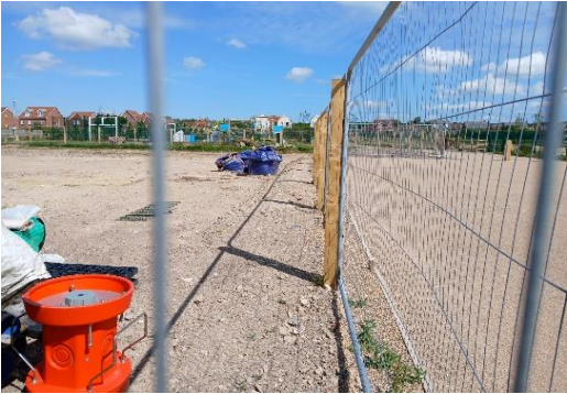
Bare ground near the entrance of the site.
