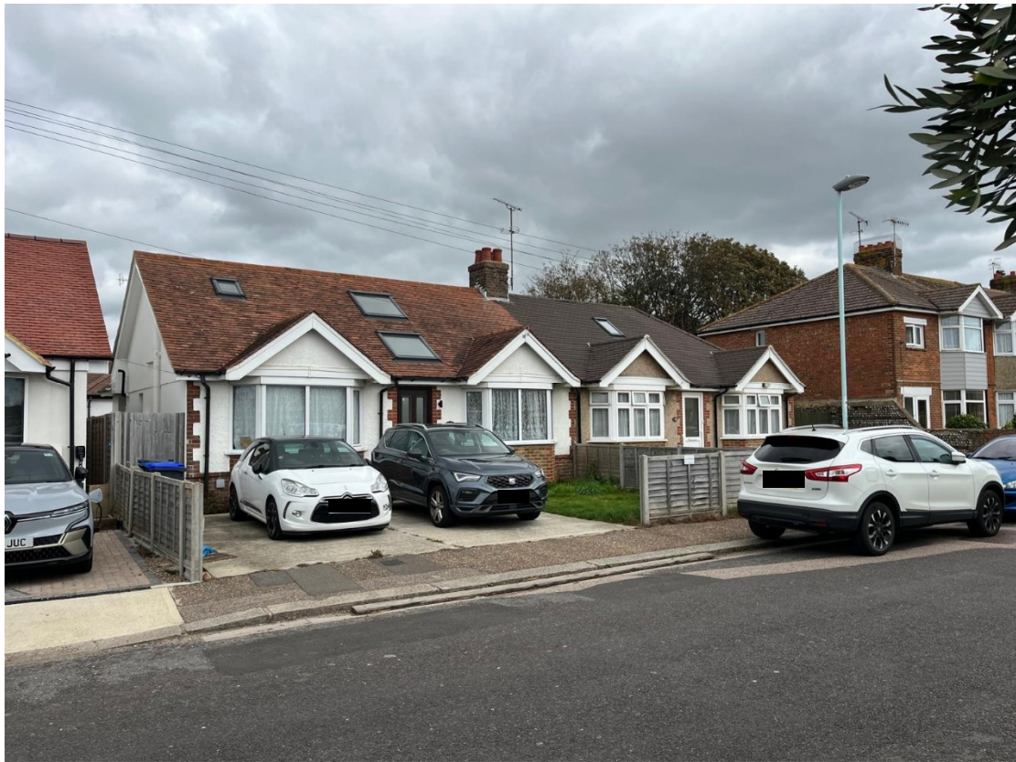
Front / south elevation showing 54 Henty Road
