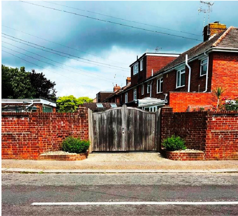
Henty Road – showing gates over 1.8m high
