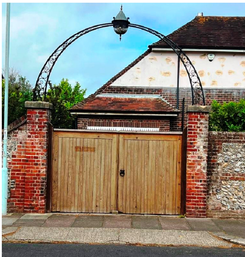
Gaisford Road – showing walls over 2m high
