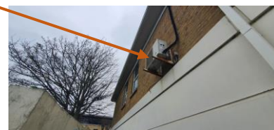
Figure 5.1.3- Existing Condenser Unit
