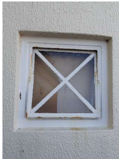
Fig 5: Typical Existing Crittall Window
