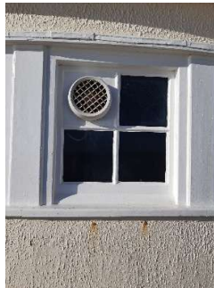
Figs 8-10: Indicative through-glass mechanical extractors showing differing types
