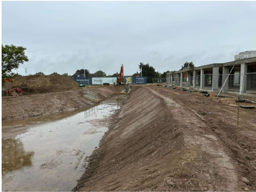
Figure 1 - Basin during construction – grading, water standing within basin
