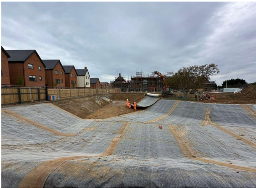
Figure 2 - Basin during construction – lining being installed
