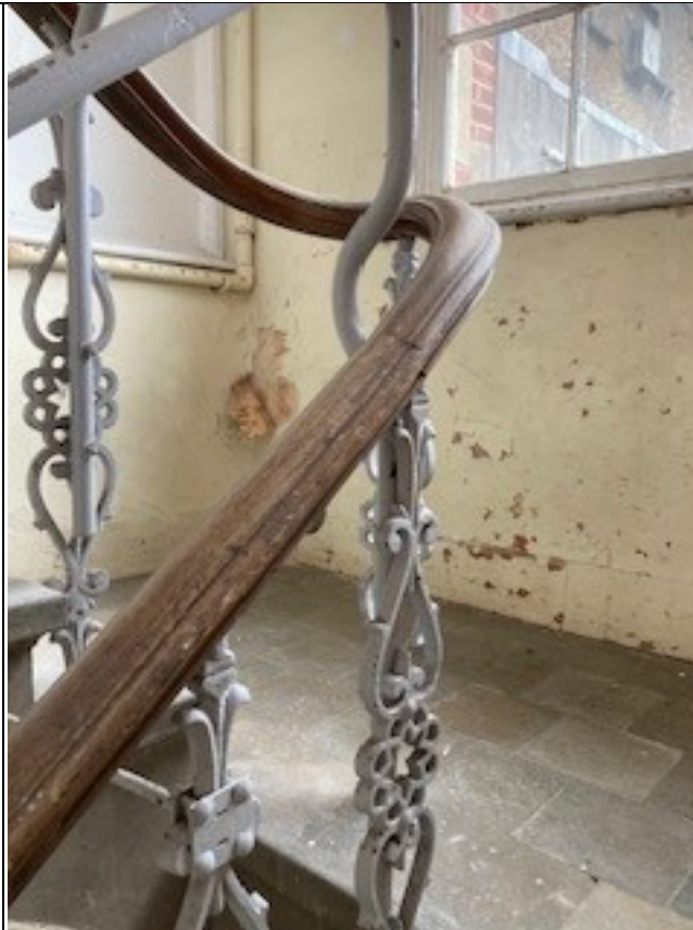
Photos 2,3,4 & 5. Interior views of New Road Stair showing the cast iron balusters and the temporary/semi-permanent cloakroom/ticket booth added later
