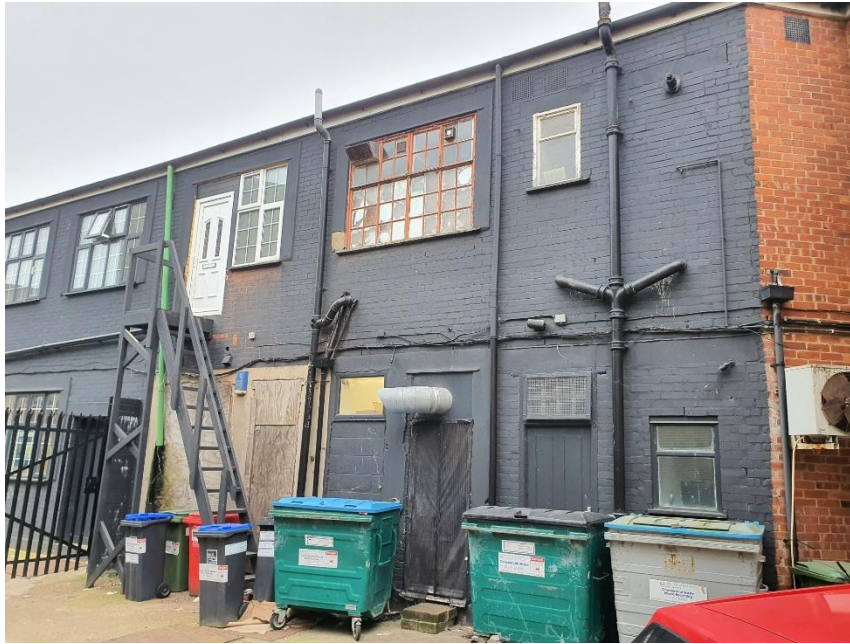
Fig. 2: Photo showing rear façade at 3-4 Liverpool buildings
