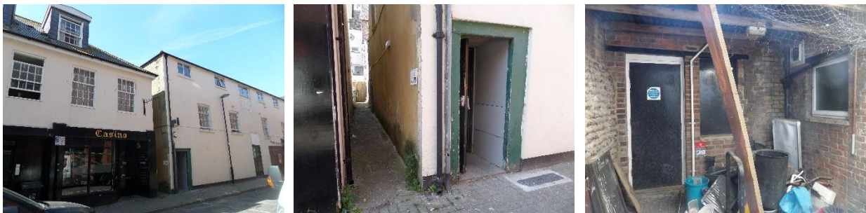
Existing access to the staircase is via an undercroft (centre photo) off Ann Street
