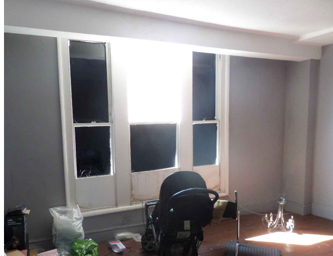
Typical internal views - Top: Dormer. Bottom: Sash window
