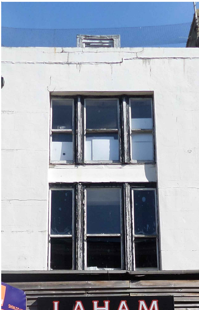
Southern windows - Refer to P018 and P019 for replacements
