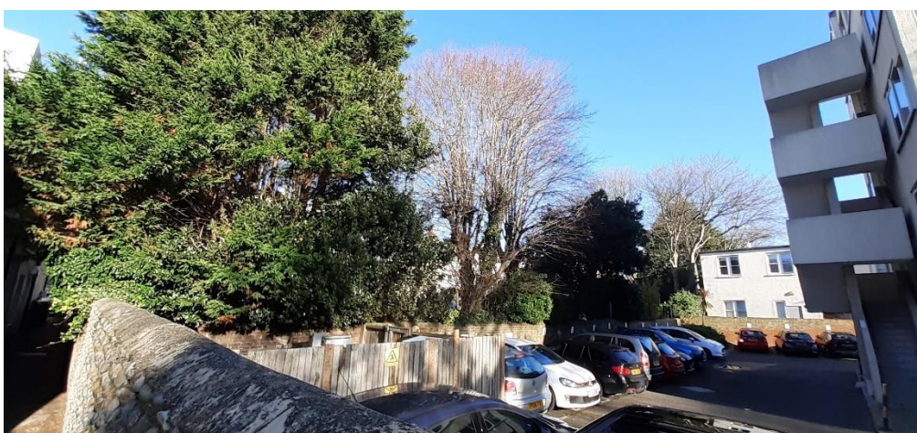
Figure 12 – Retaining wall, Southfields House car park and sub-station
