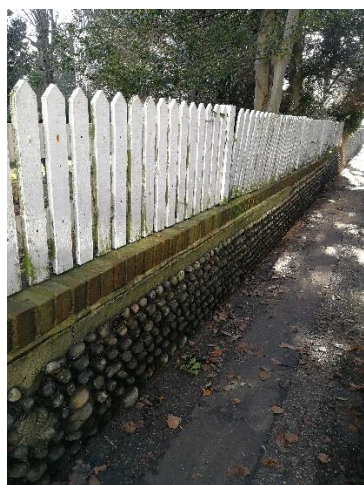
Figure 13 – Reduced flint wall
