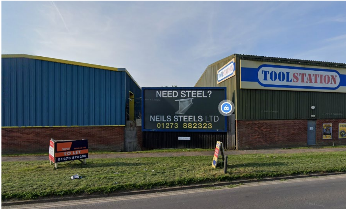
Figure 1: Streetview of the subject site.
