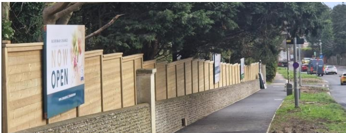
Figure 1: Temporary signs on front wall (looking south-east)
