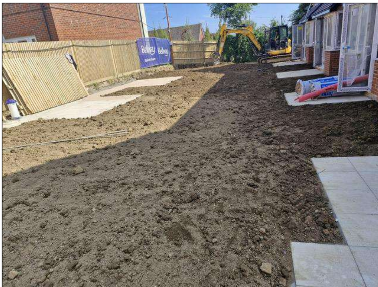
Figure 5-C: Laying of topsoil (contractor provided)
