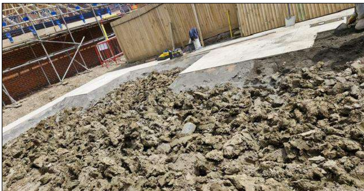
Figure 5-B: Laying of subsoil (contractor provided)
