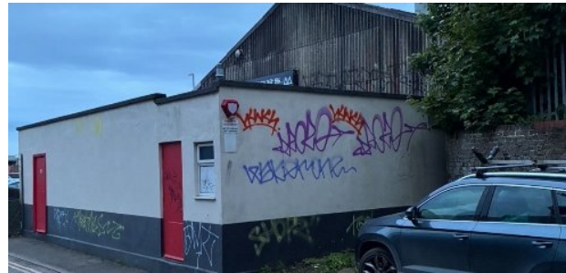
V1 B1-2 surveyor photo
