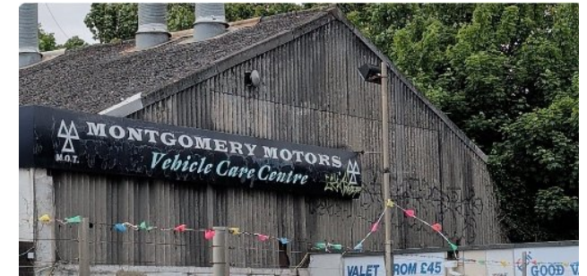
V1 B1-3 surveyor photo
