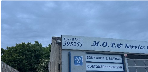
V1 B1-1 surveyor photo
