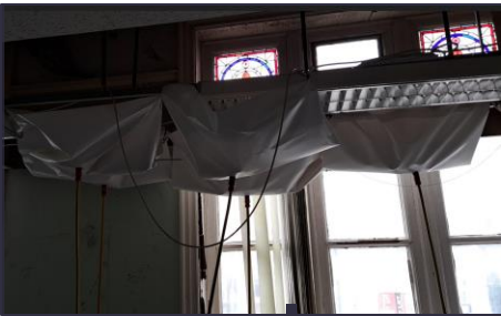
Water ingress appears to have been remedied. Leak occurs beneath Thord floor level roof voids. Roof survey required to determine remedials.
