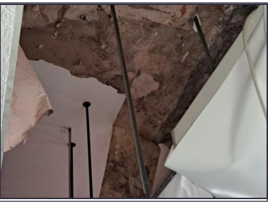
Water ingress appears to have been remedied. Leak occurs beneath Thord floor level roof voids. Roof survey required to determine remedials.
